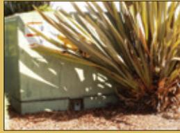
from AMP's main distribution lines to a usable level for your home and your neighbors' homes. From time to time, AMP's crews must gain access to these devices for maintenance or for restoring power.
