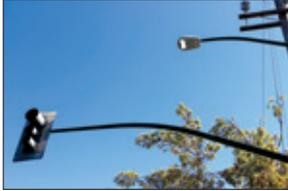
LED street lights last longer than high pressure sodium lights—about 12 years compared to 5.5 years—thereby significantly reducing maintenance costs. LED lights provide much better illumination and color distinction at night, while reducing sky glow—the artificial illumination of the night sky.
